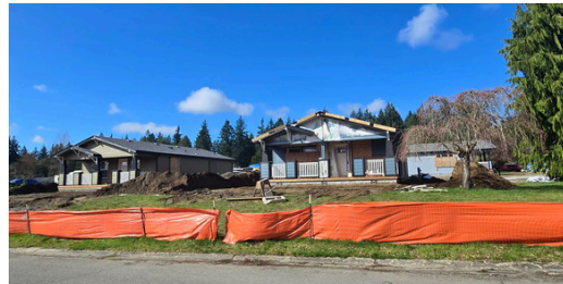
New Units installation progress
